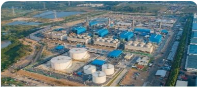
Gas-fired Power Generation
